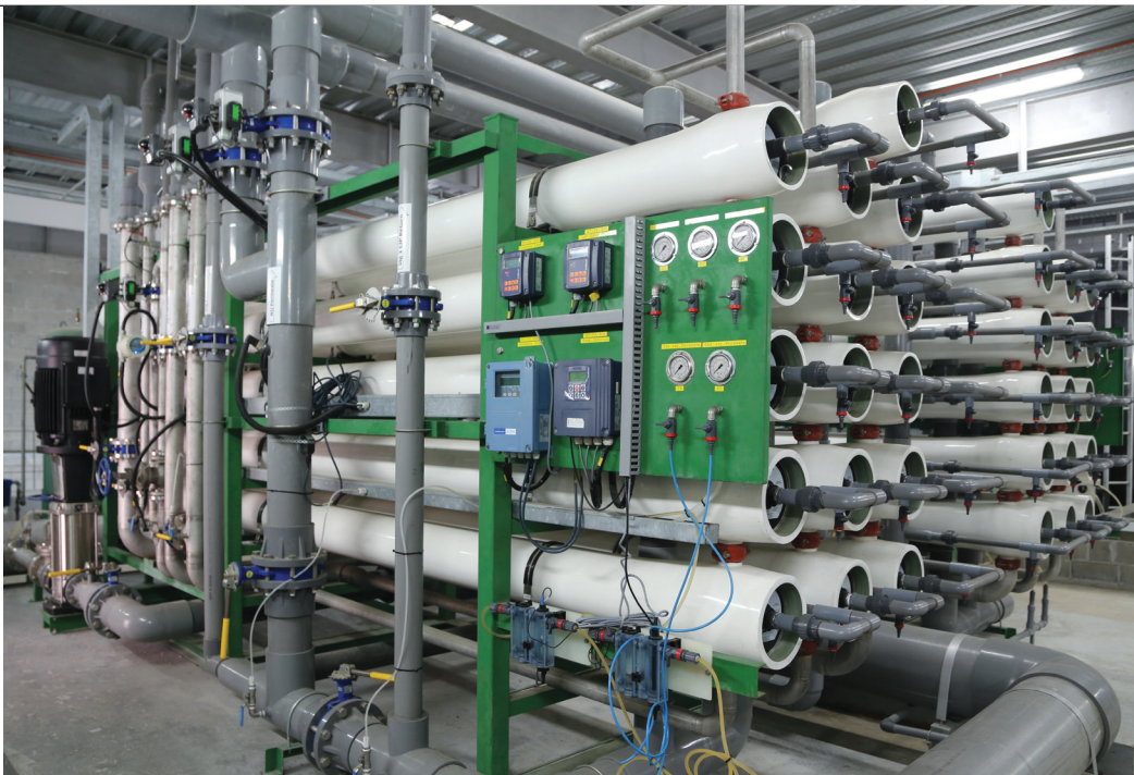
The water treatment plant in Sunway South Quay will use the water in the existing South Quay lake to produce approximately 10,000m³ of water a day to serve a host of commercial buildings in Sunway City.
